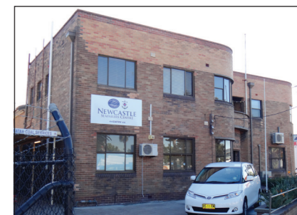
External view of the Seafarers' Centre, Newcastle.
